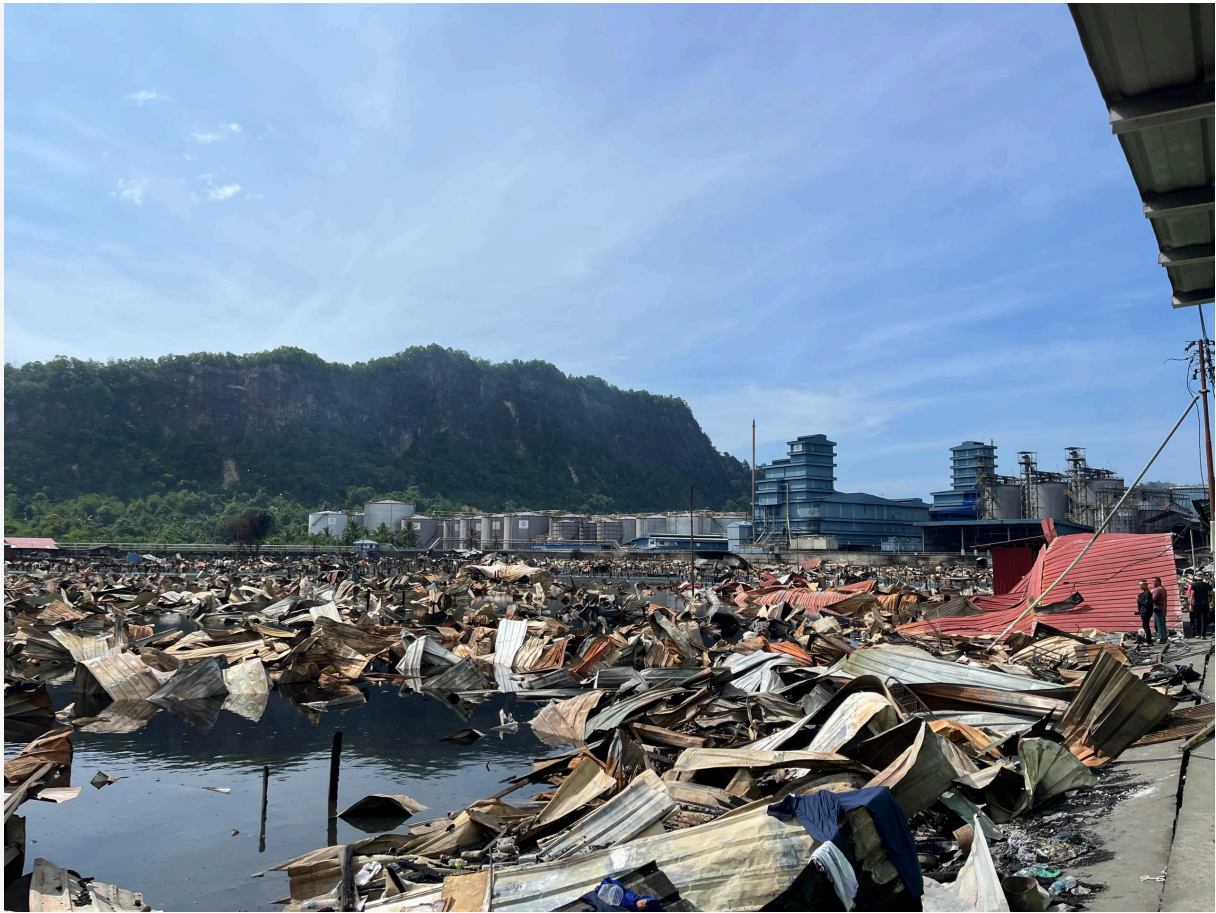
Large-scale housing destruction in Kampung Bahagia. (Photo: MRCS)
