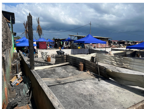
Temporary shelters amid fire-damaged structures. (Photo: MRCS)
