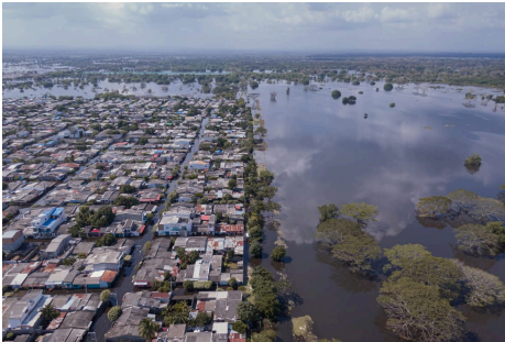
Flooding in the municipality Montería, Córdoba. February 2026.
