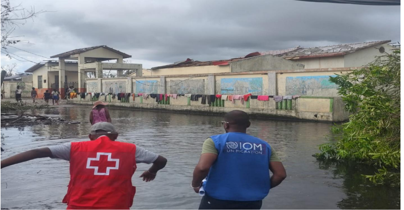
Destruction of houses in Toamasina by Tropical Cyclone Gezani, with the MRCS supporting joint assessments. (Photo credit: MRCS)
