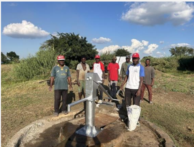
CVM volunteers and community members demonstrate the use of a newly rehabilitated handpump, restoring access to safe water for flood-affected communities in Gaza Province.
