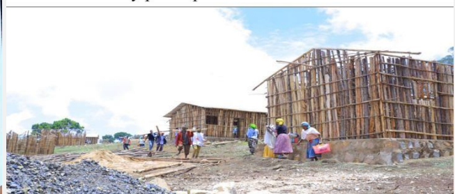
Community participation in shelter construction
