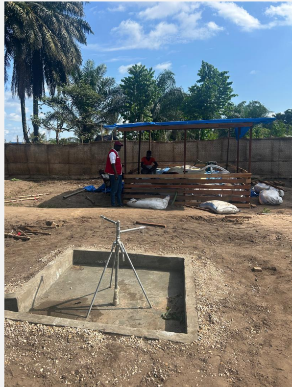
Installation of bladers at the camp base of Bulape - Photo: IFRC
