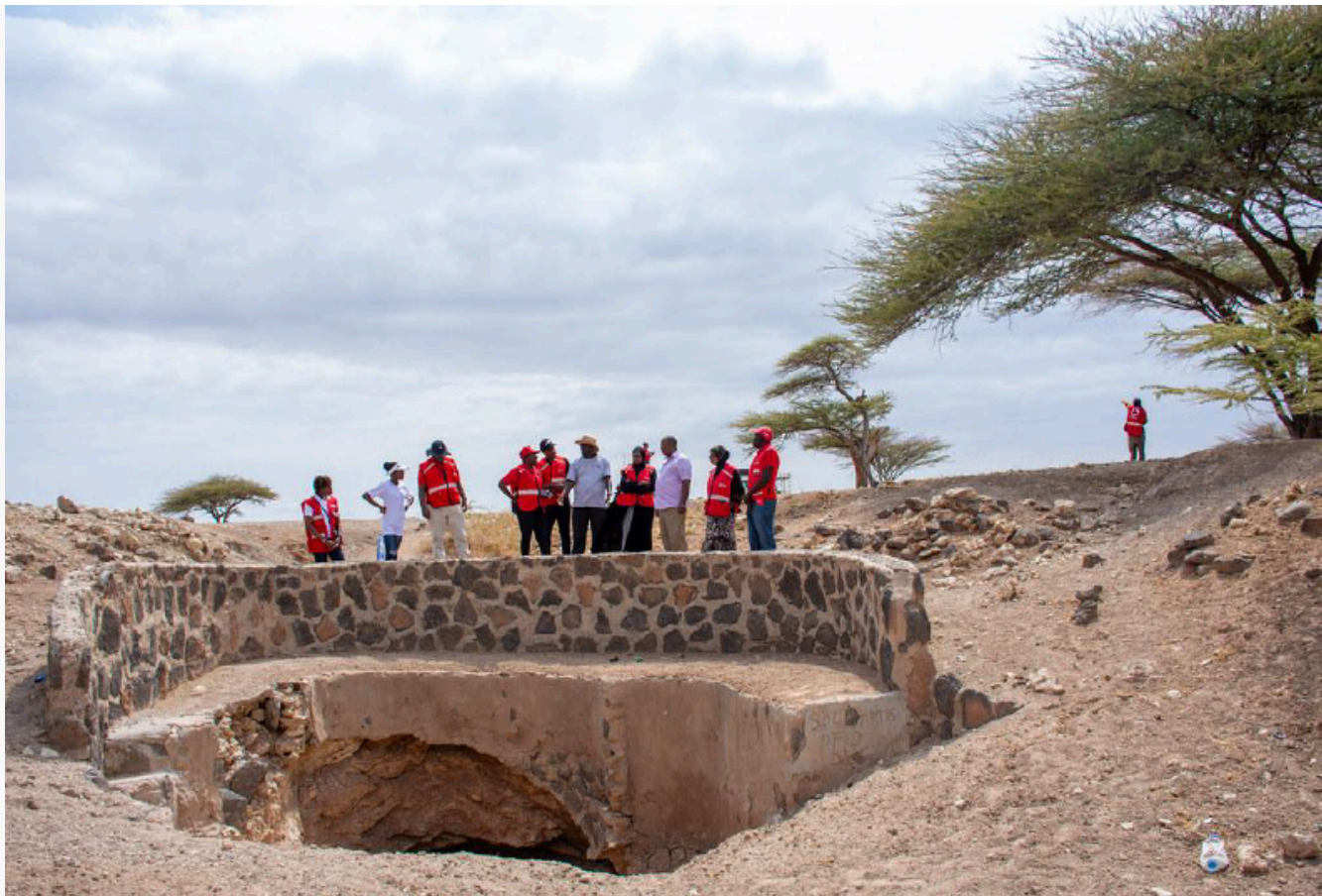
KRCS inspect a dilapidated dry water point @Marsabit- drought assessment.
