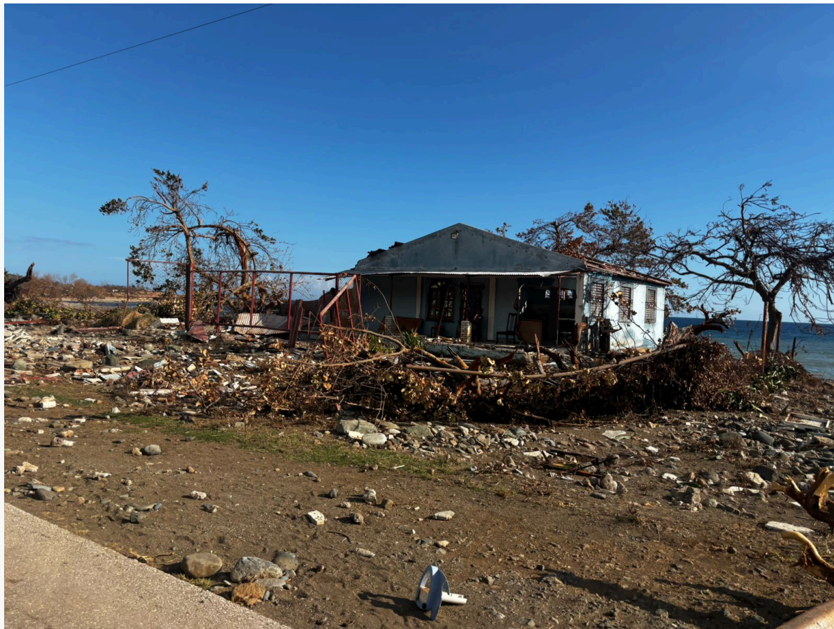
House Destroyed in the Municipality of Guama. Santiago de Cuba. IFRC 2025
