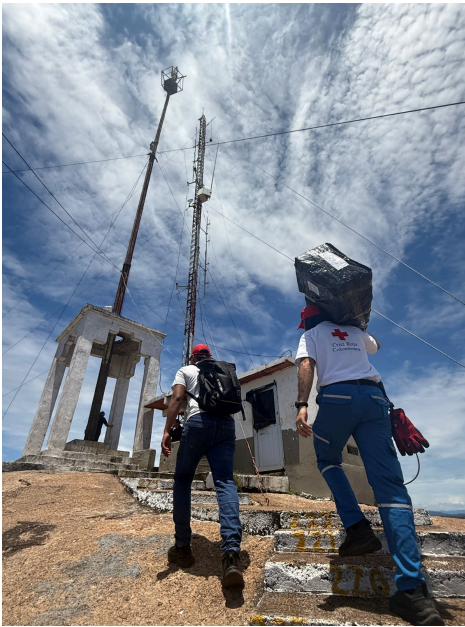
Maintenance of the National Society's local telecommunications network.
