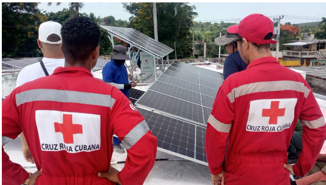
Installation of photovoltaic system in Jiguani Hospital, Granma Province, July 2026. Source: Cuban Red Cross.
