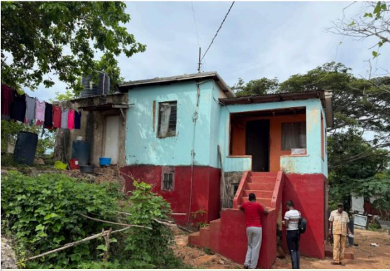
A home being assessed for the shelter rehabilitation programme © 2025 Jamaica Red
