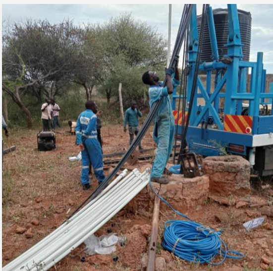
Ongoing works during a borehole rehabilitation in Isiolo
