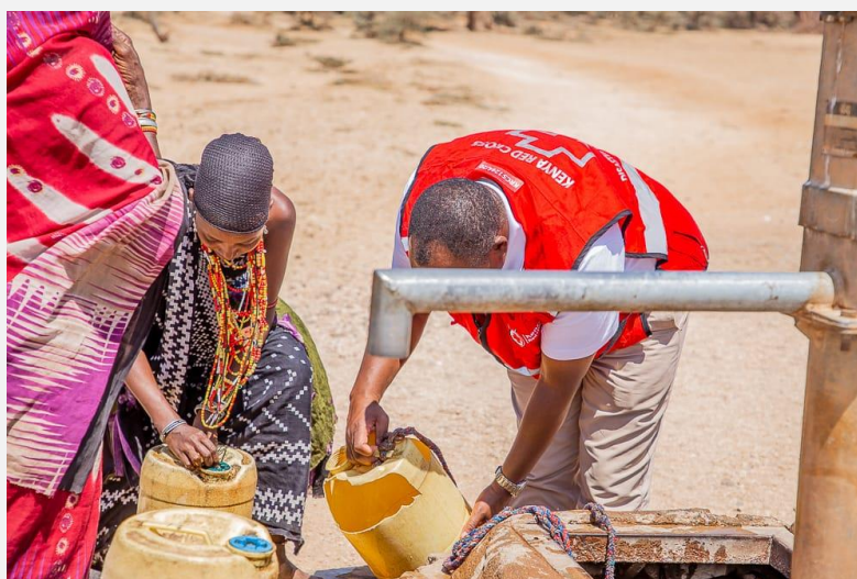
A hand pump borehole in Marsabit
