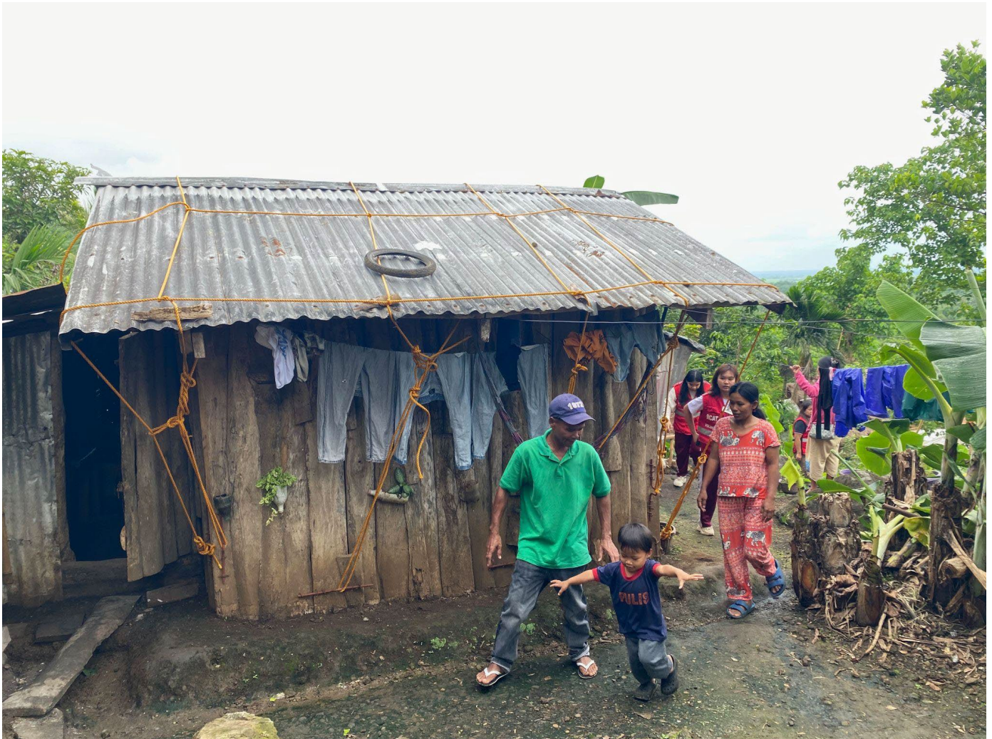
Shelter strengthening kits installed ahead of STY Uwan in Isabela remained intact a month after the activation. (Photo: IFRC)
