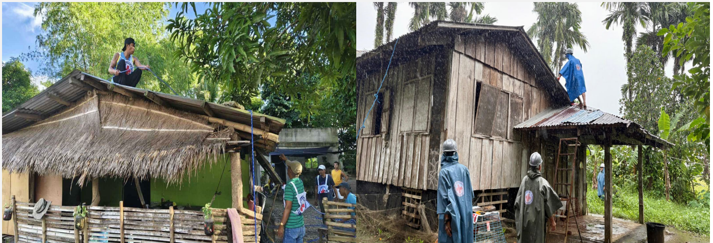
Installation of SSKs in Isabela and Quezon provinces. (Photo: PRC)
