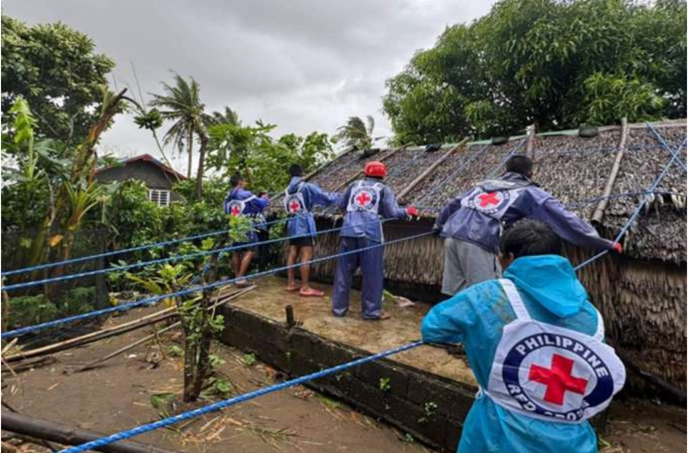
Installation of Shelter Strengthening Kits in Villa Leonora, Buguey, Cagayan as part of Typhoon Marce Activation on 6 November 2024. (Photo: PRC)
