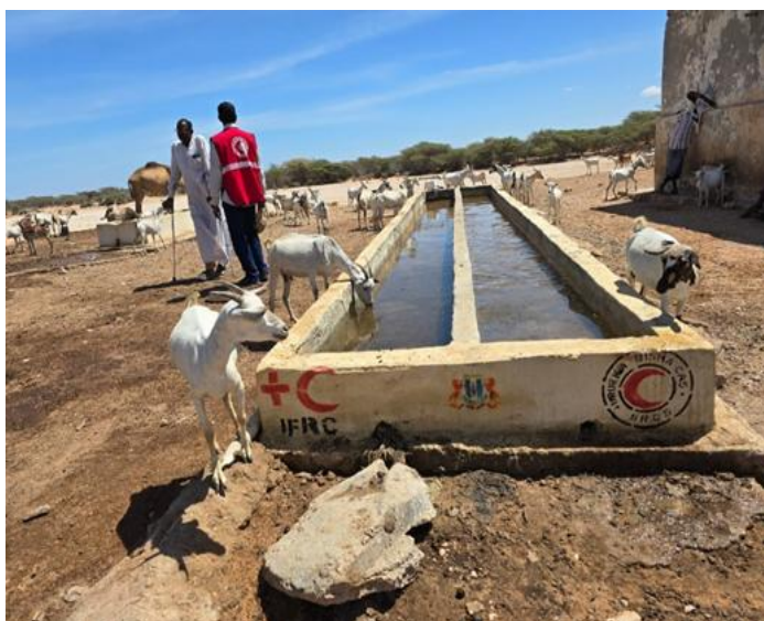
Figure 2: A water trough constructed for the livestock to access sufficient water
