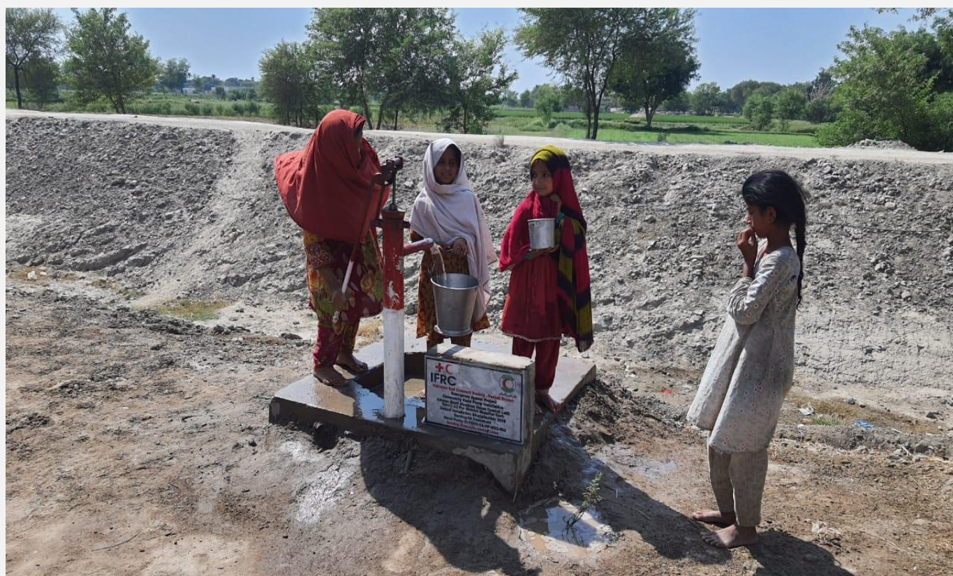
Children collecting water from the newly constructed handpump in district Muzaffargarh, Punjab (Photo: IFRC, Country Delegation)
