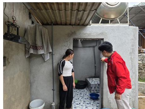
New latrine in Nghe An Province (Photo: VNRC)
