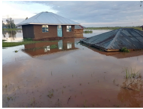
Destroyed household by the ongoing floods
