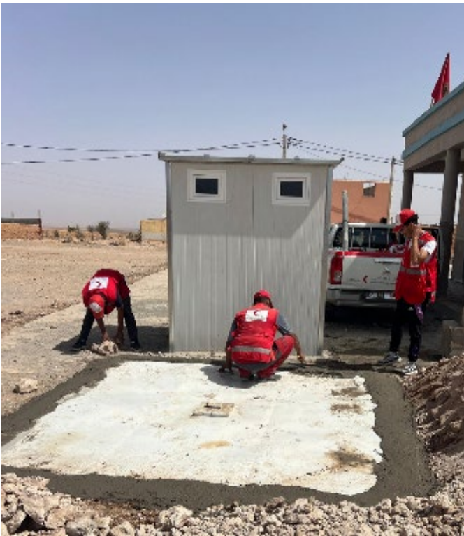
Photo - Installation of toilets modules in El Haouz (September 2025)
