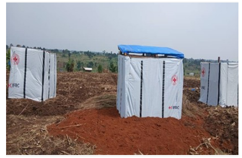
Emergency bathrooms and latrines constructed in Nakivaale
