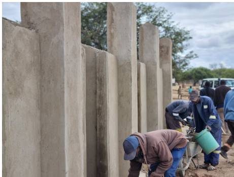
Construction of disability and girlfriendly latrines
