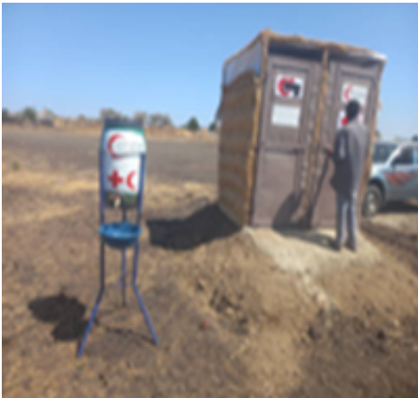
Sanitations installed with latrines and handwashing in one affected areas
