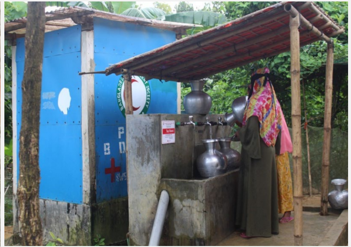
Displaced households in camps 11, 18 and 19 collect safe drinking water from solar powered water networks, conveniently available next to their shelters. (Photo: BDRCS)
