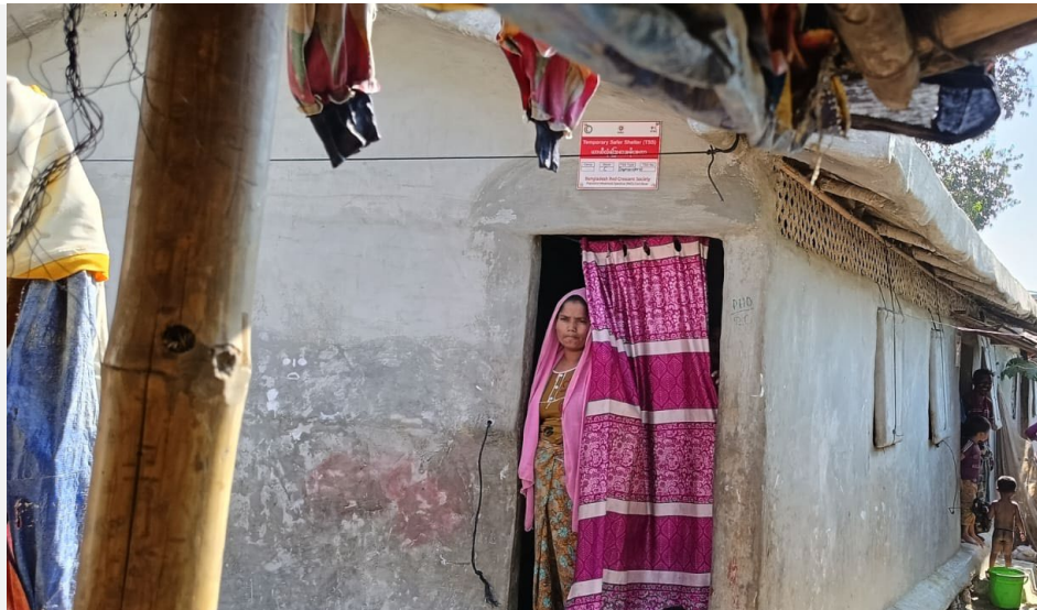
The newly constructed upgraded shelters already in use by households in Camp 11 and 12. The households expressed utmost satisfaction acknowledging its special fire, weather and extreme heat resilient features. However, to replicate this design in entire camps is subject to fund availability, while existing mid-term shelters being used and repaired. (Photo: IFRC)
