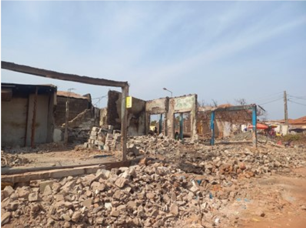
Gabú Central Market Fire incident, Guinea-Bissau
