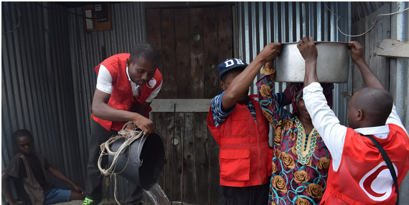
The Comoros Red Crescent supporting communities by restoring water tanks after cyclone damage (Photo: IFRC)
