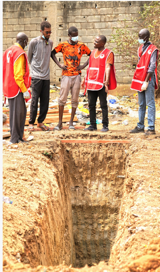
facilitated access to water and sanitation in Juba and Aweil refugee centers by installing water tanks and bladders, mobile latrines
