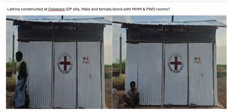
Latrines constructed at Dalakara IDP site
