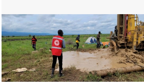
Borehole Drilling works by the contractor with supervision from URCS WASH
