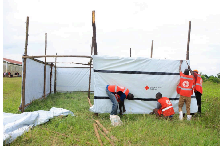
URCS volunteers setting up temporary shelters
