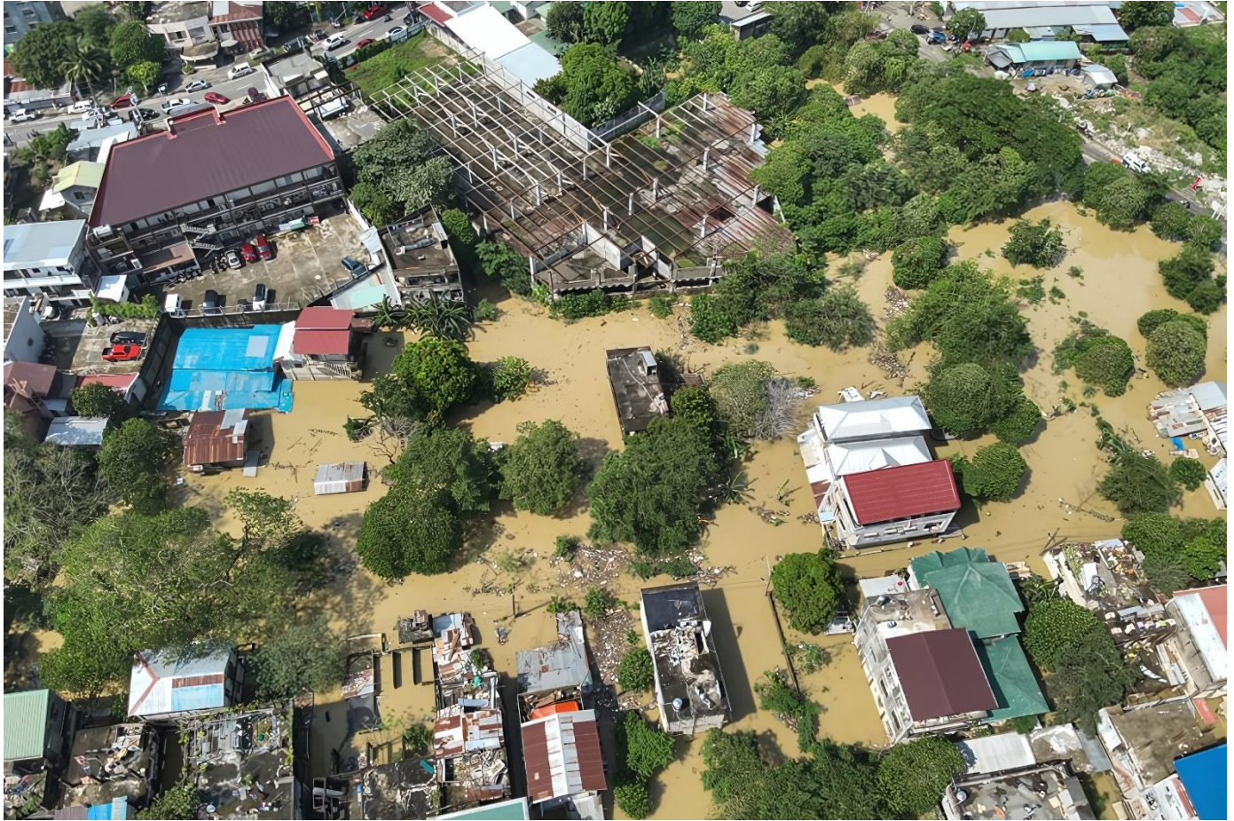
Aerial shot of the high flood levels impacting the community in Tuguegarao, Cagayan. (Photo: Cagayan Public Information Office)
