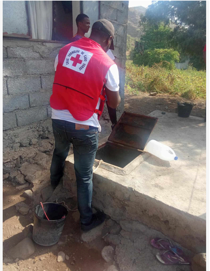
Disinfection of a water tank
