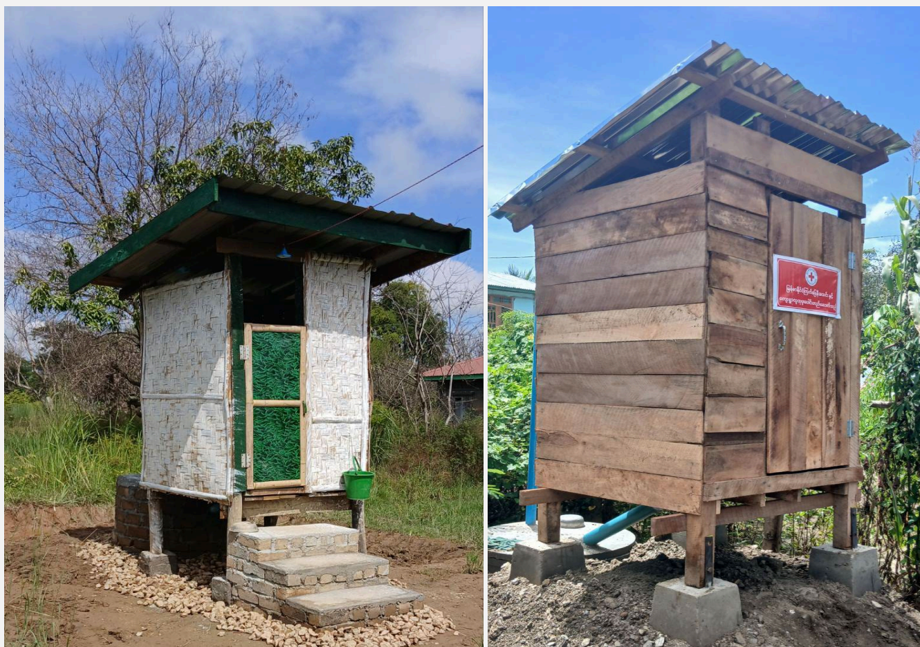
MRCS provided standard latrine designs to affected communities, including a concrete sanitation pit and elevated flooring to improve safety and hygiene. Communities were able to use locally available materials based on their preference and access. Left: bamboo sheet walls. Right: wooden walls. (Photo: IFRC)
