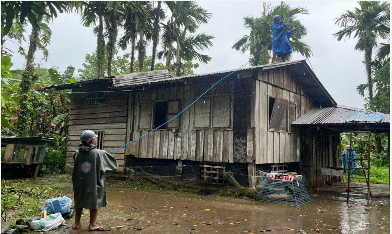
Installation of SSK in Quezon province. (Photo:PRC)
