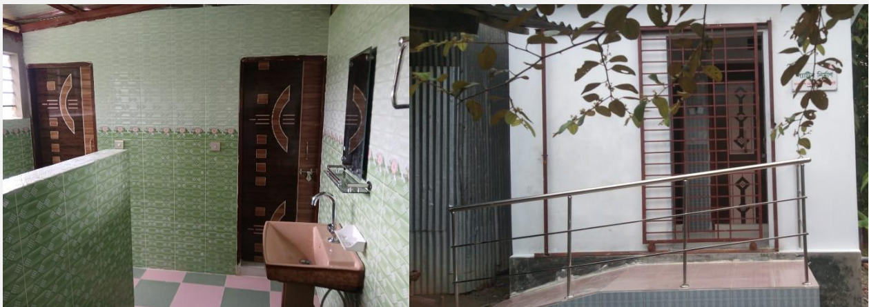
Constructed WASH block in Shamser Gazi High School, Feni (L) and Darul Ulum Mohammadia Mohila Madrasa in Lakshmipur (R) (Photo: BDRCS)
