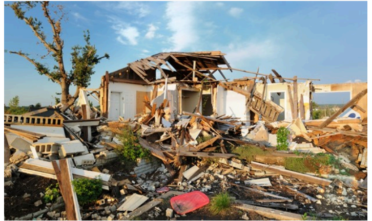
the picture above shows damages in the Tongaat area of KwaZulu Natal in South Africa
