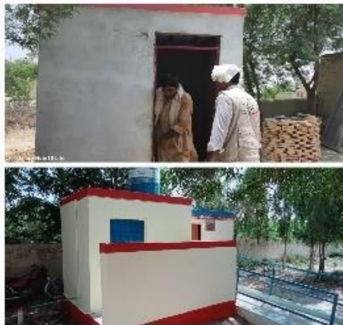
Improved WASH facilities in BHU Khairpur (Photo: PRCS)
