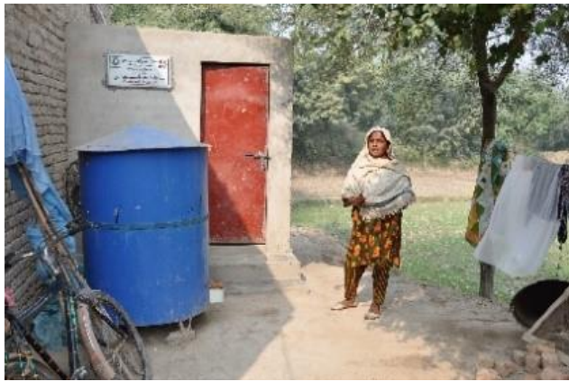
Latrine construction brought safety and dignity to Shama Khatoon and village women, ending years of risk. (Photo: IFRC PMER)
