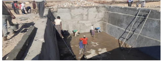
Figure 4: Rehabilitation of a berked in Somalia
