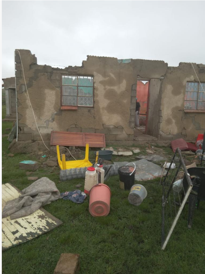
Totally destroyed by storm surge in KwaZulu Natal Province
