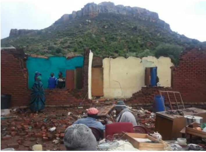
Totally destroyed house following storm surge coupled by strong winds that occurred on the 22-28 December in Quthing District. Source LRCS
