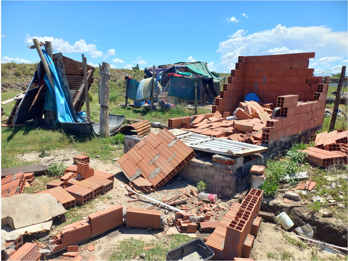
House destroyed by the storm. Bahía Blanca - Source: ARC.
