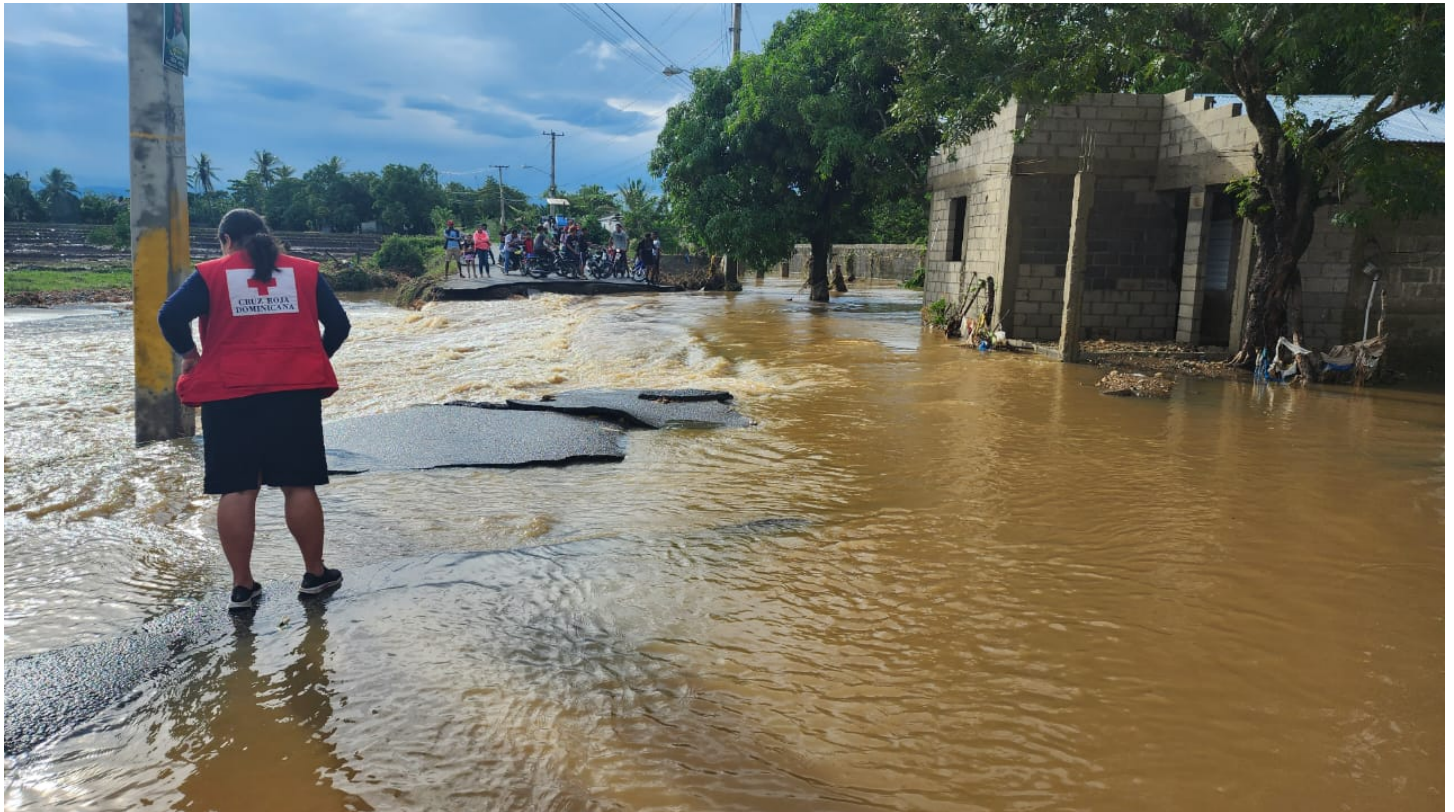
Bridge collapse on the community of Cuca, Duarte province.
