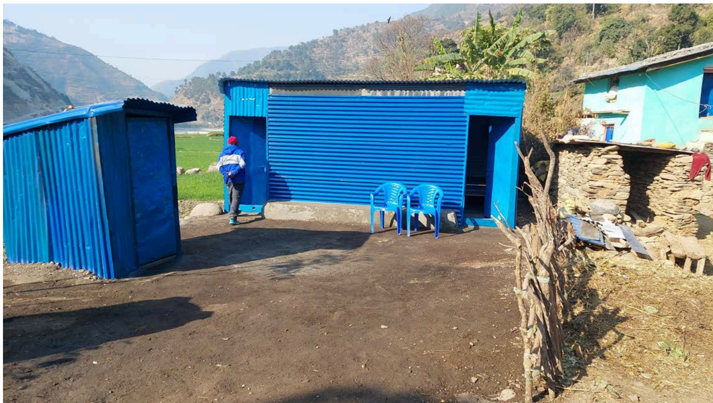
Newly constructed transitional shelter with toilet in one of the affected districts. (Photo: NRCS)
