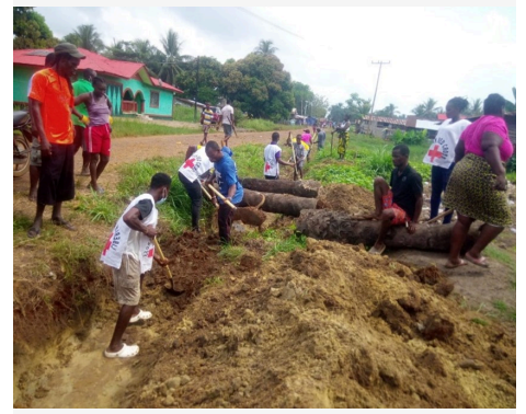
Cleaning of drainages by volunteers and community members
