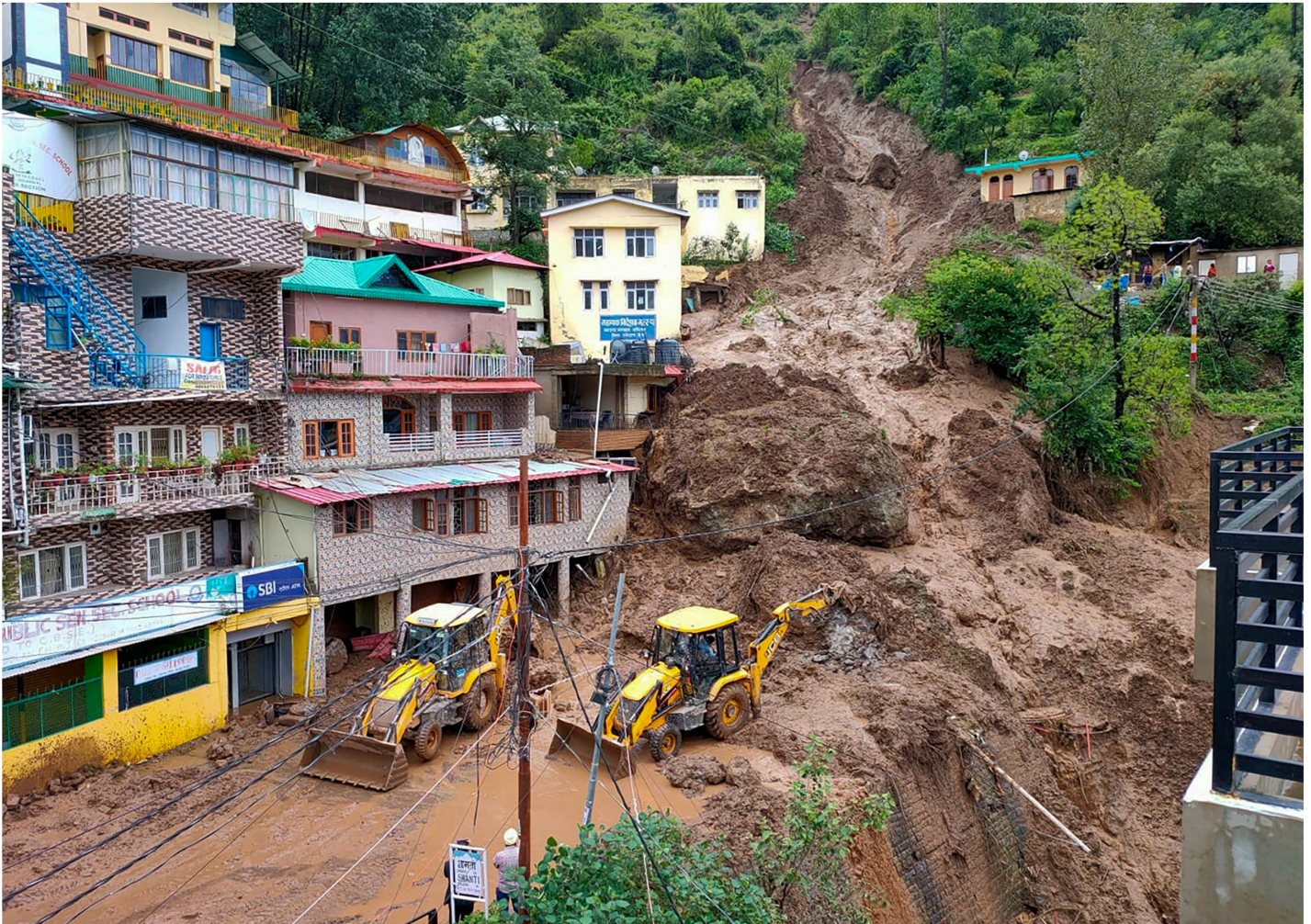
Destruction in Manali by Heavy rains and landslide. Pic: Business Today Newspaper
