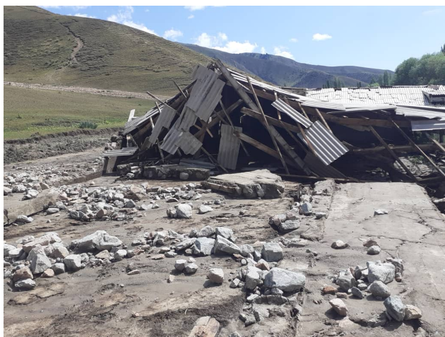
Damage caused by the mudflows. Photo credit: RCSK.
