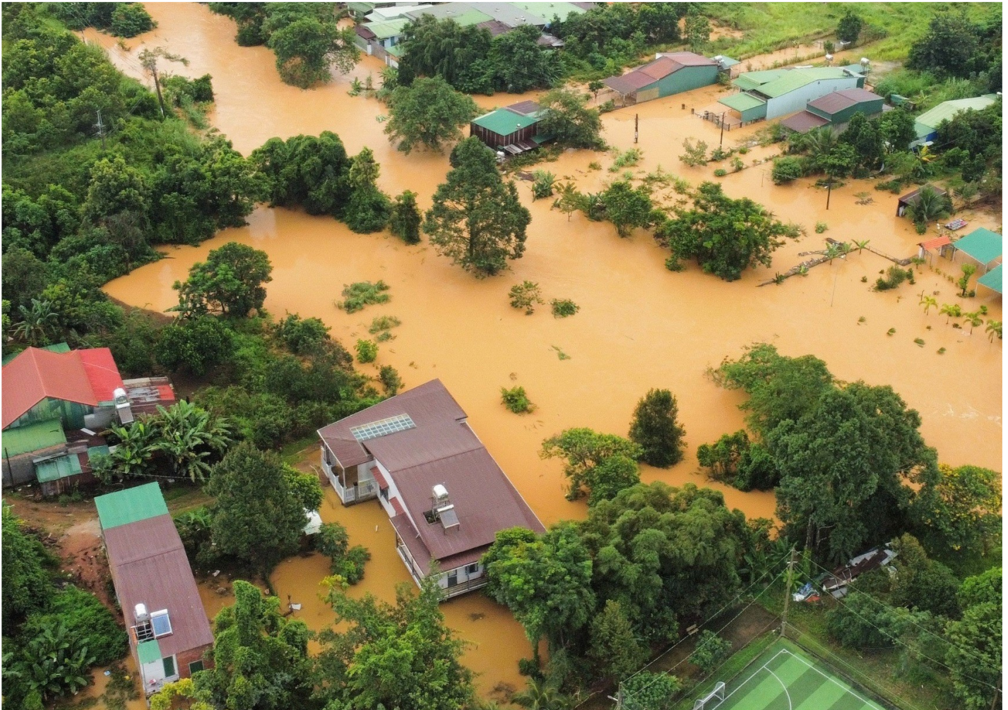
Aerial view of the affected areas. Houses are inundated by flood waters (source: media)
