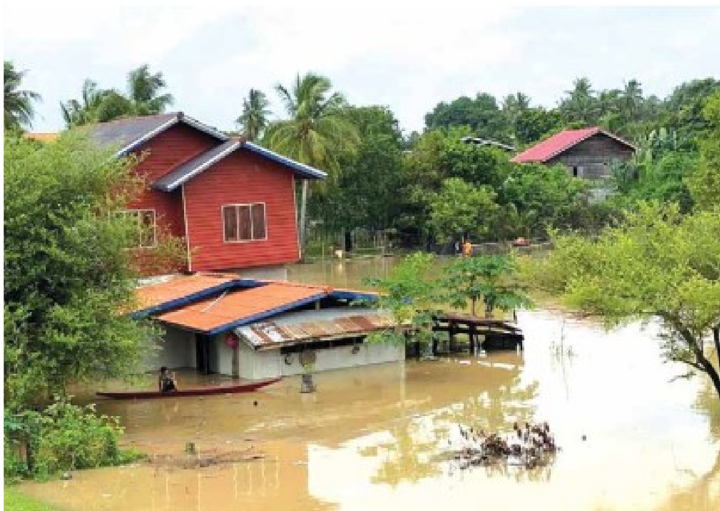
Damaged house in Savannakhet Province (Photo: Pathelao daily)
