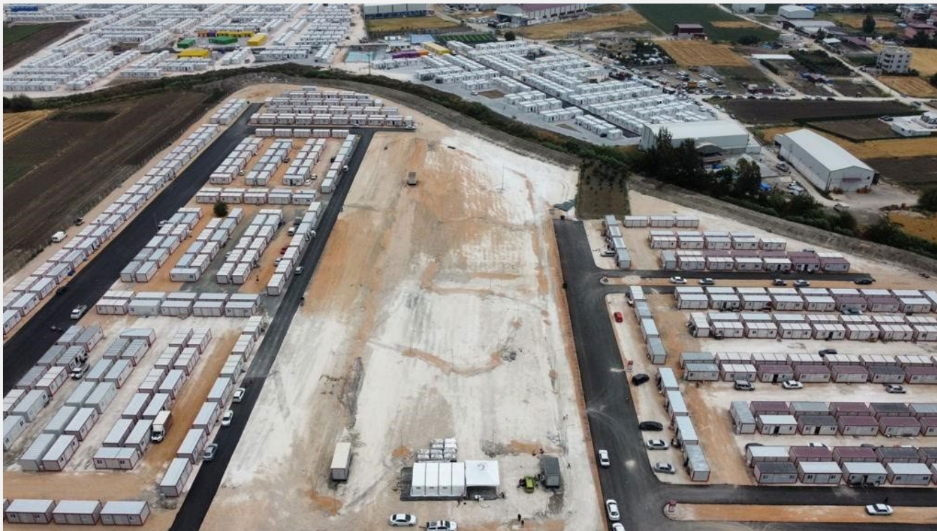
Aerial view of a container camp settlement in Hatay. Photo credit: IFRC, July 2023.
