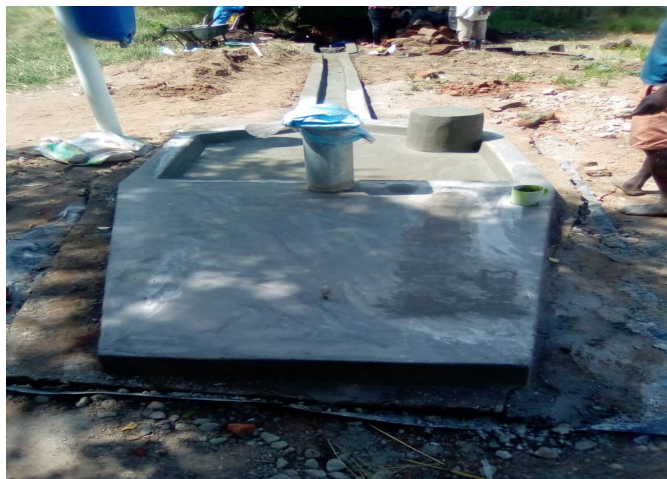
Borehole rehabilitation in progress in Salima
