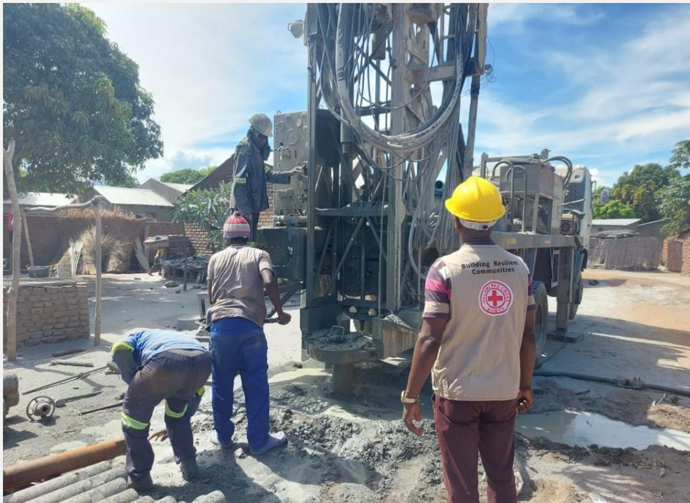
Borehole drilling in Nkhatabay
